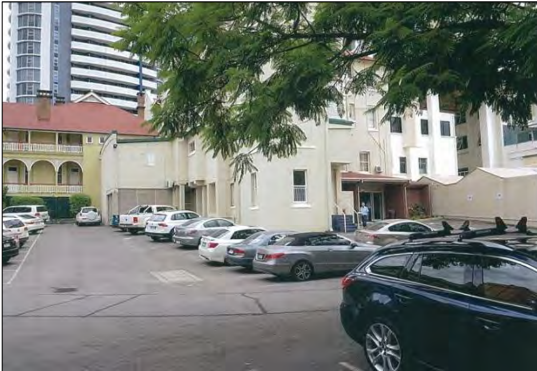
The painting depicts a view from the early 1990s. A close comparison with the 2017 photo reveals the major changes to the buildings. Note the changes to the verandas and rear of the Green House, the extensions for the new kitchen and connections between the buildings, the new rear entry and lift, the removal of the old outbuilding on our boundary to the right of the rear entrance, and the changes to the background due to the new high-rise buildings.
