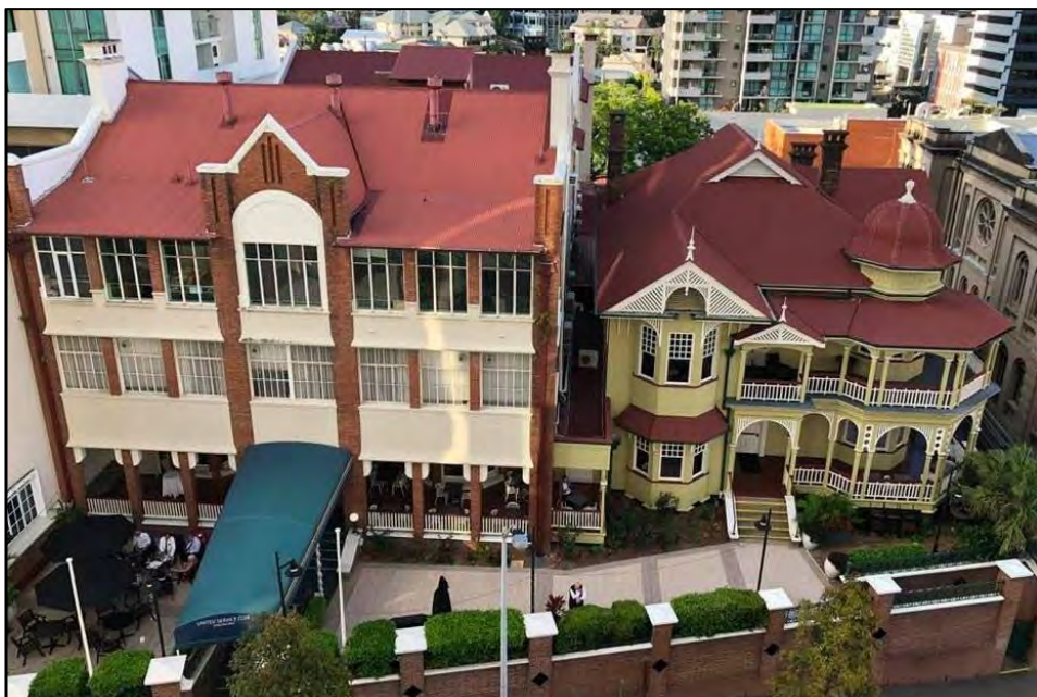
Nov 2017. The extension and connection works of mid 1990s are clearly visible.
